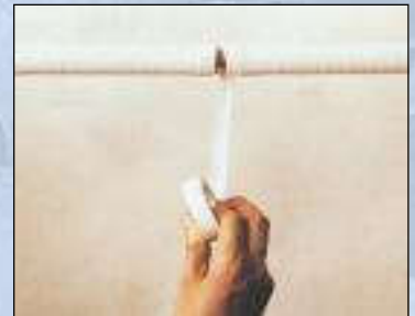
When the joint is complete and cool, fold back the plastic coat and wrap the joint to give continuity of protection.
